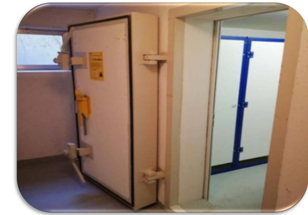
Turning basements into emergency shelters
